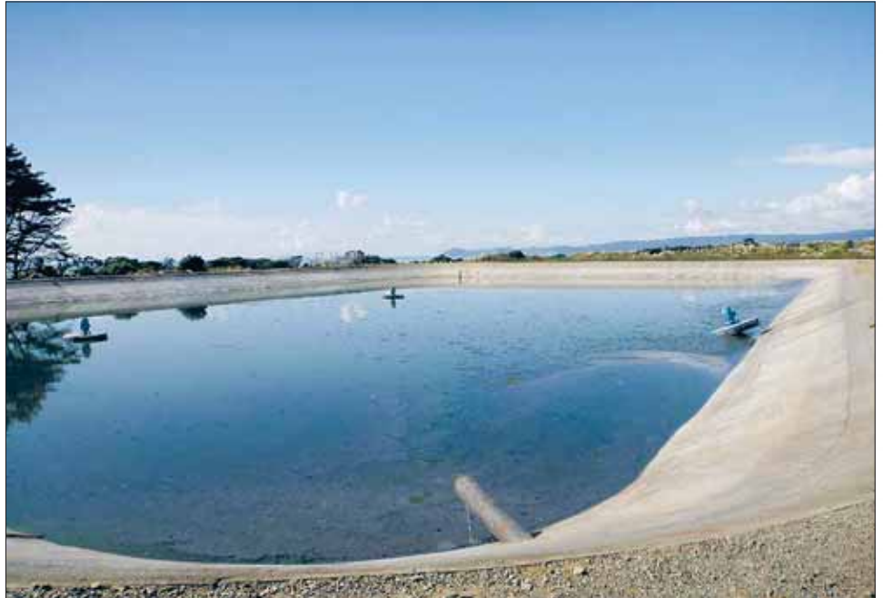
The Waipu Wastewater Treatment Plant is also located in the dunes
