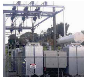
Old transformers from the 1950s and 1970s, supporting up to 2500 homes and businesses. On the right - New 10MVA transformers, capable of supporting up to 5000 homes and businesses.
