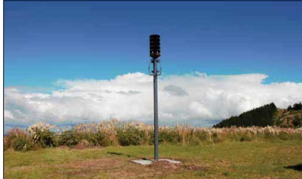
The first new siren partially installed in the Whangārei port area.
