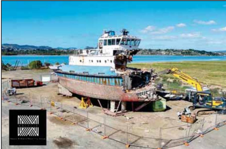
Northport recently commissioned Marsden Metals and Waste to decommission and recycle their end of life tug.
