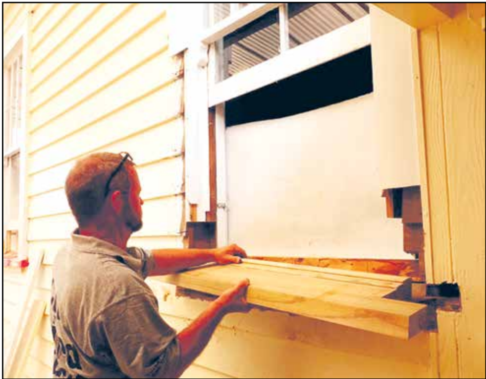
Carpenter Steve Sparkes from John Land Builders fitting a new window sill on the Coronation Hall to replace some rotten timber.
