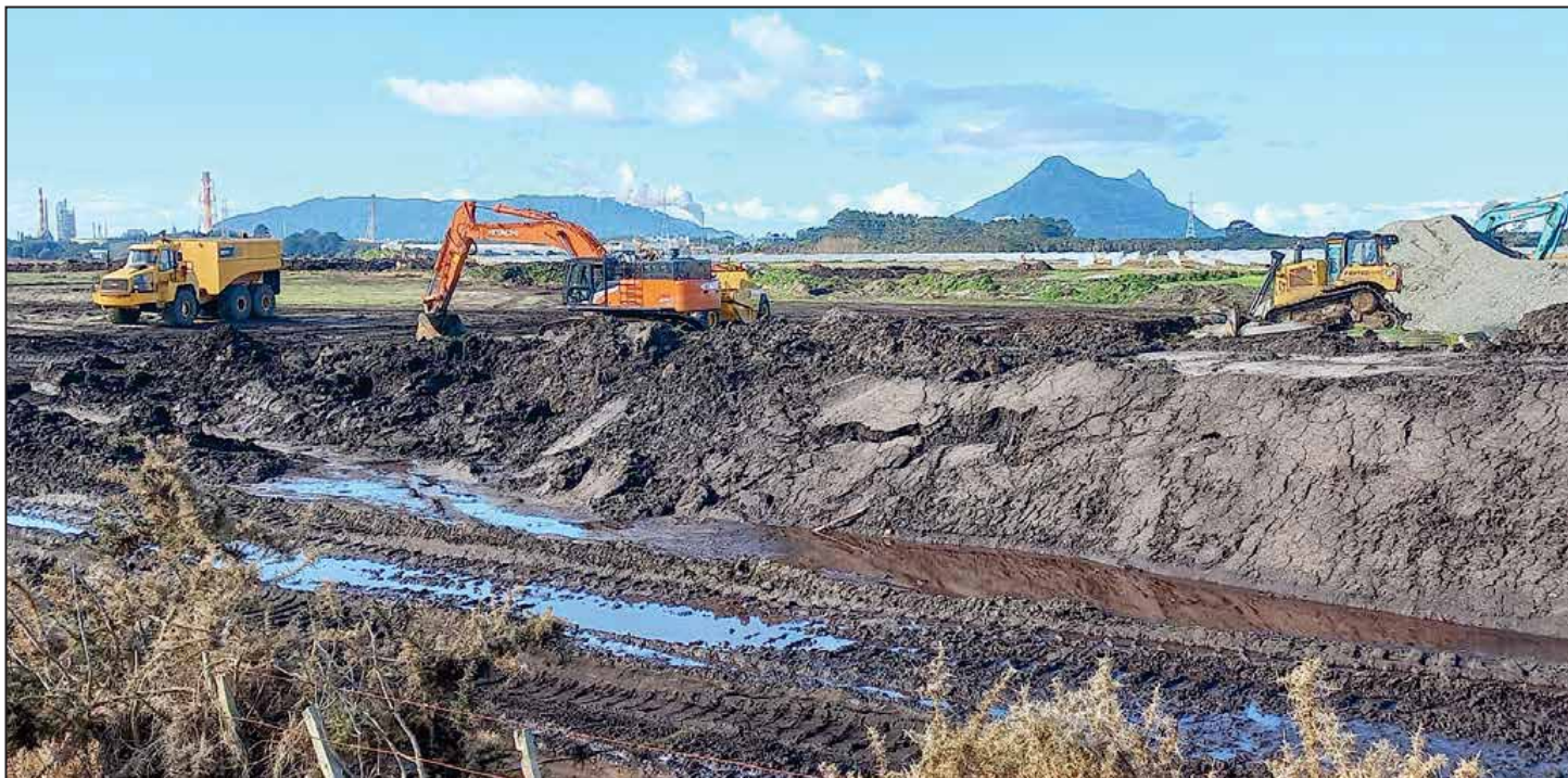
Site preparation for solar panels taking place near the Port Marsden Highway and Marsden Point Rd. intersection
